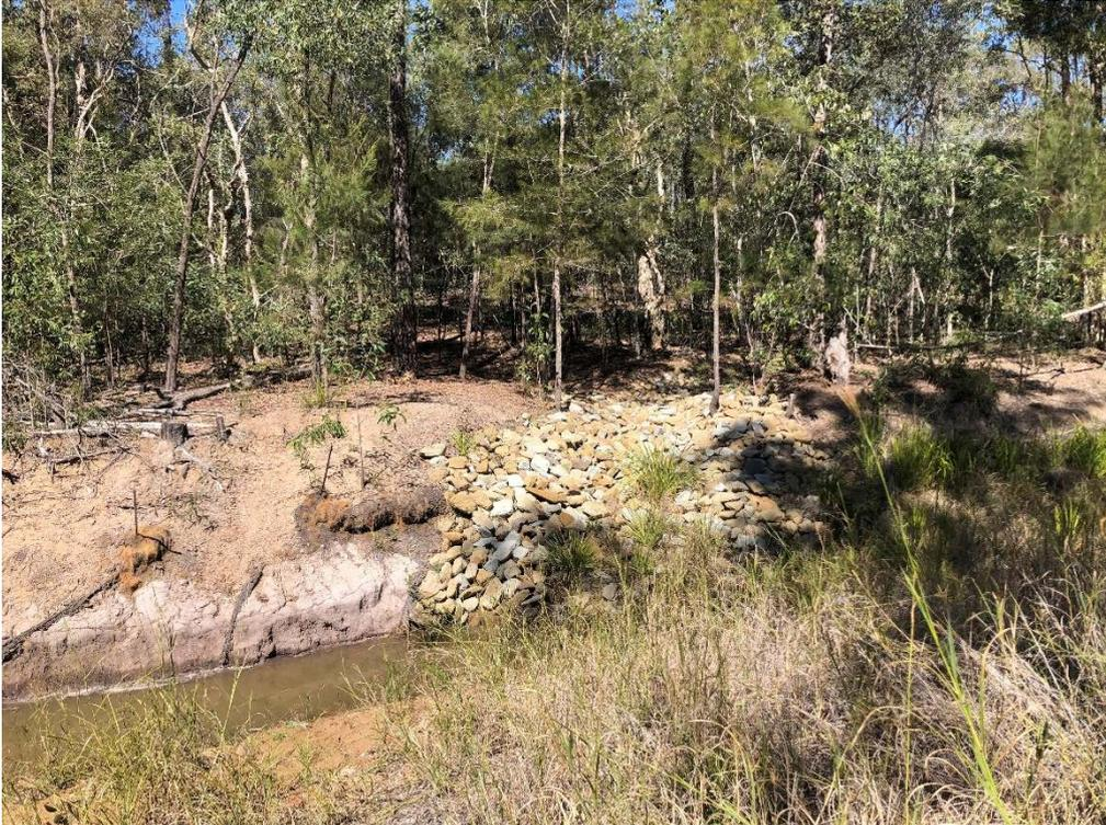
**Photo 10: Rocks installed to assist in protecting topsoil and reducing erosion from overland flows into tributary.**
