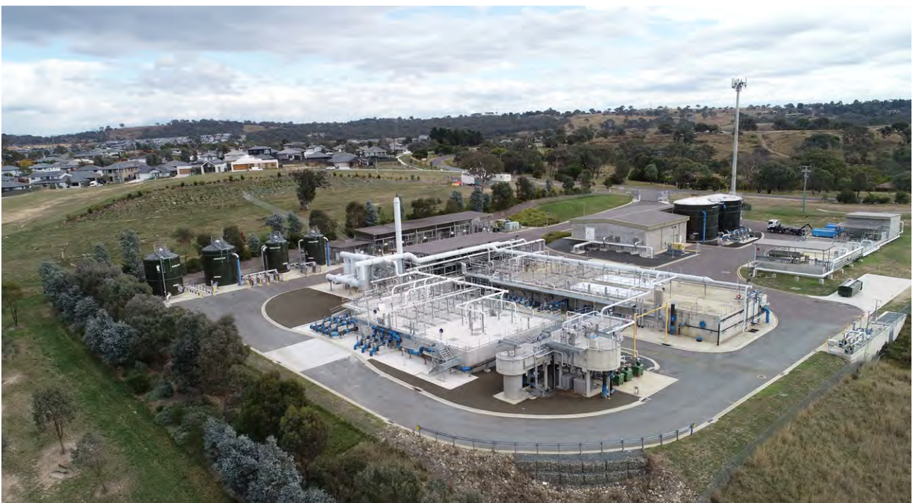
Googong Water Recycling Plant
