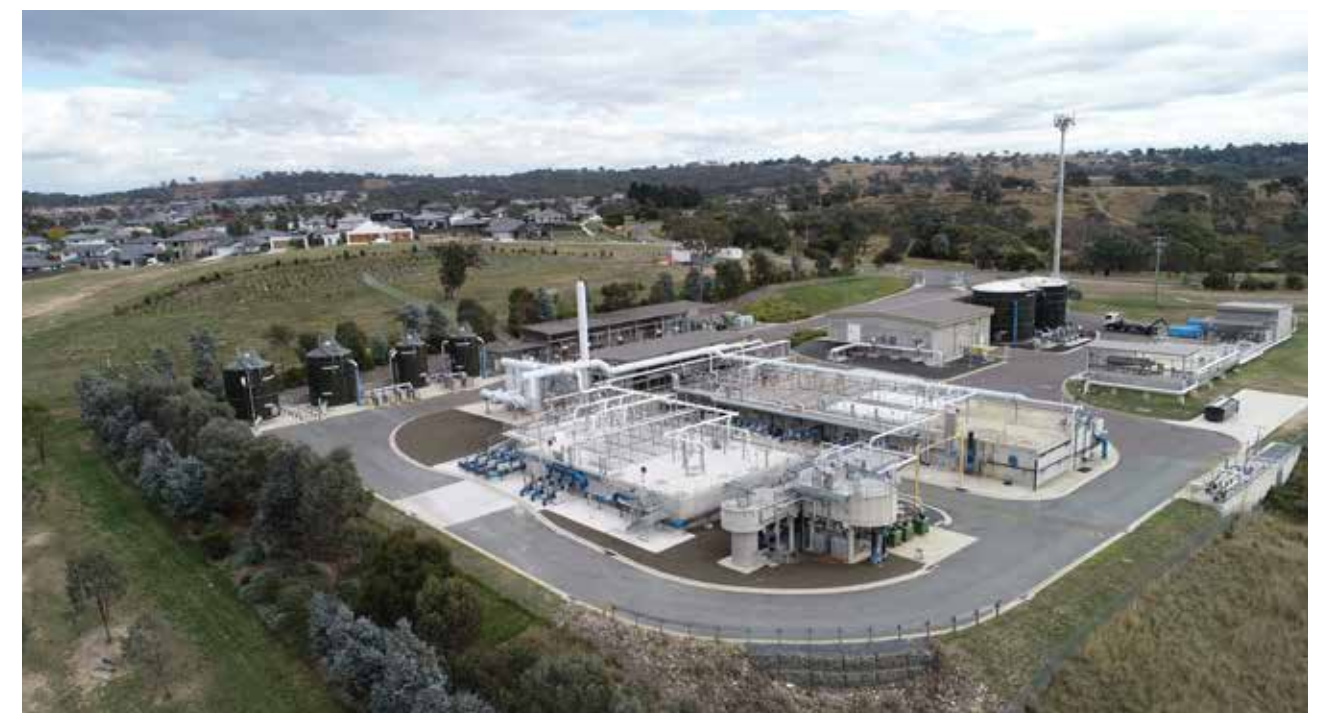
Googong Water Recycling Plant
